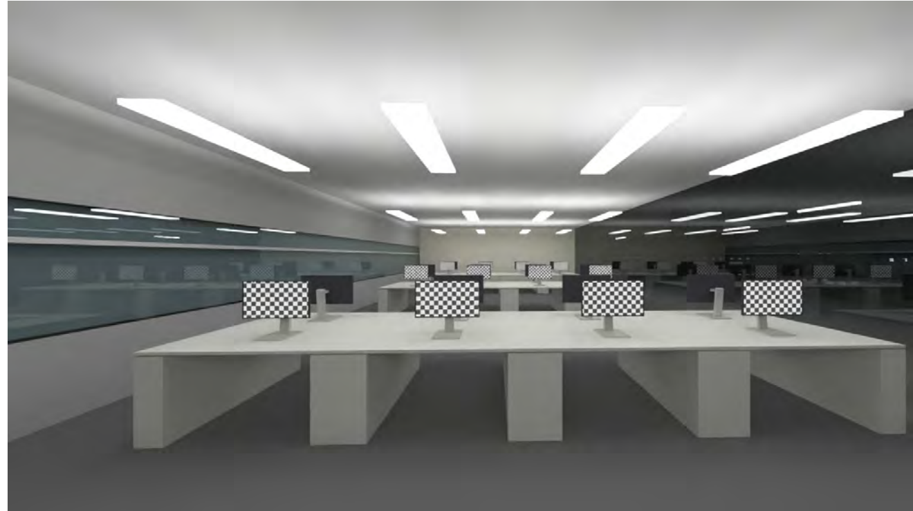
Final Design: Direct/Indirect Lights in the working space
